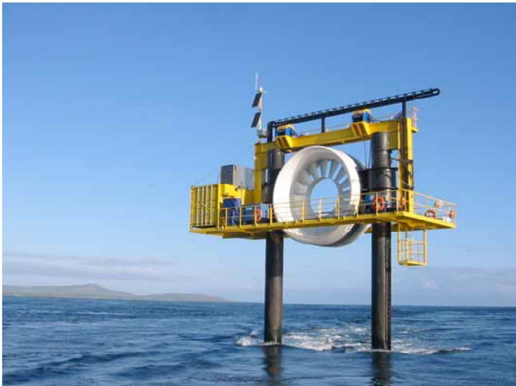
**Figure 1:** OpenHydro Turbine at Fall of Warness site (EMEC)
