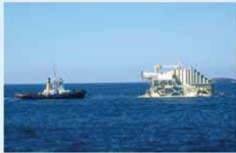
MK1 Full scale evaluation unit (fixed to seabed)
